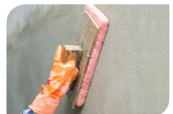
Sponge the external surface for a texture finishes. 第二步用海绵洗出沙粒墙面。
