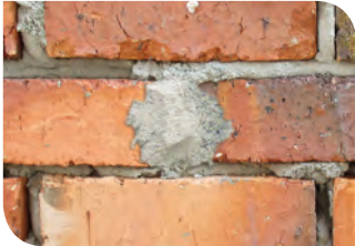
Mark required thickness with level pegs. 用灰饼标记所需的厚度。
